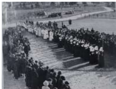
Left & right- further scenes from the laying of the foundation stone in October 1935. Note the market gardens in the background. At the right is Lady Huntingfield and Sister Ida.
